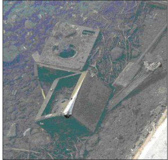
Fig. 12 Washing machine in intake channel
