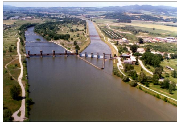
Fig. 4 WS Trenčianske Biskupice – weir and intake structure of intake channel for HPP Kostolná
