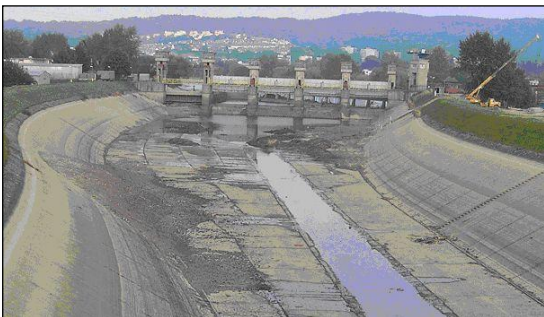
Fig. 7 Sediments behind intake structure Trenčianske Biskupice
