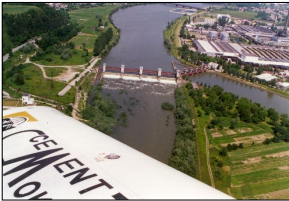
Fig. 1 WS Dolné Kočkovce – weir and intake structure of the intake channel for HPP Ladce
