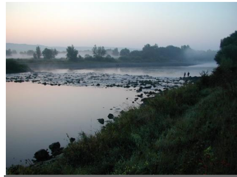
Fig. 4 The chute at the end of the HPP Madunice outlet channel (downstr.view)
