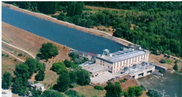
Fig. 3 The hydropower plant Madunice
