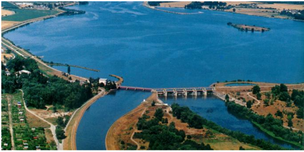
Fig. 2 Intake structure of HPP Madunice intake
