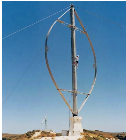
Fig. 5b Darrieus wind turbine
